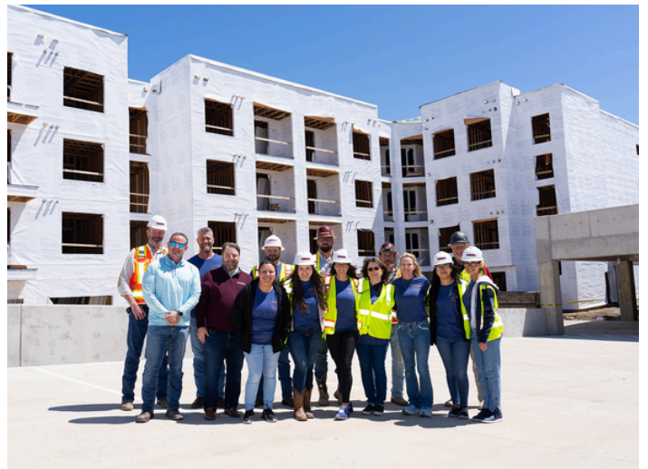
Above: The KWA team after Caroline Eastside Apartments topping out celebration in Richardson, Texas
